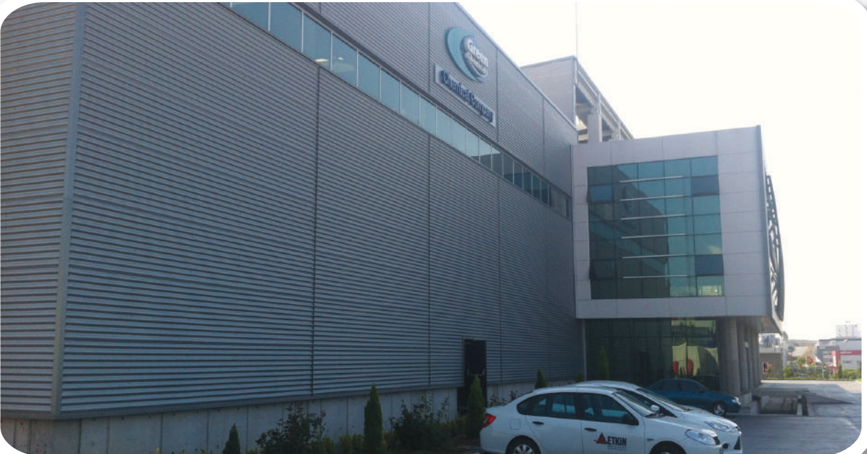
Green Chemicals Gebze Fabrikası mekanik tesisatı. Mechanical installations of Green Chemicals Gebze Factory buildings.
